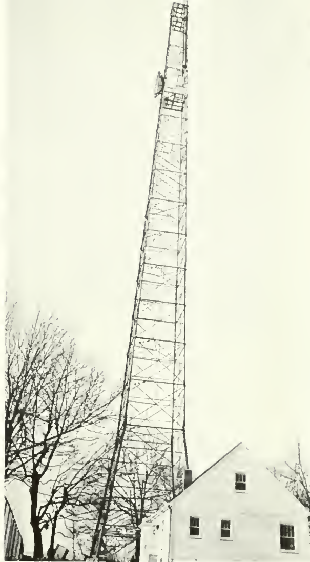
THIS 210-FOOT TOWER SUPPORTS THE ANTENNA IN NBC'S UHF EXPERIMENTS.
